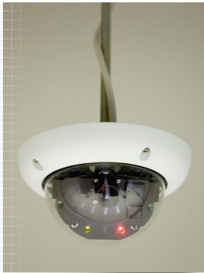
The implemented solution is a system with voice and video surveillance cameras mainly composed of Mobotix MX-D24, which cover the entire space area.
